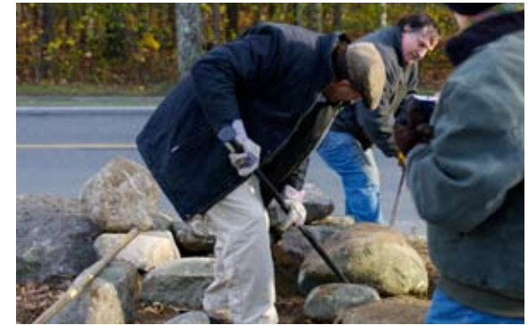
Robert Young of New England Stonemasonry and Buzz Constable use pry bars to move a large boulder at the Garden Club's workshop.
